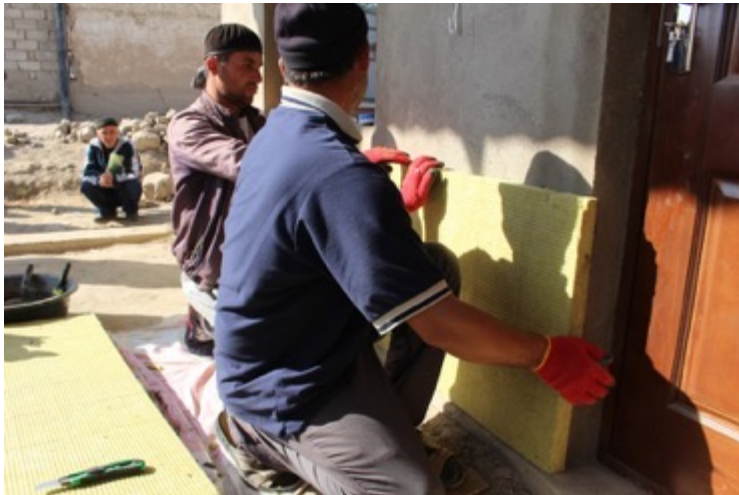
Insulation of exterior walls
