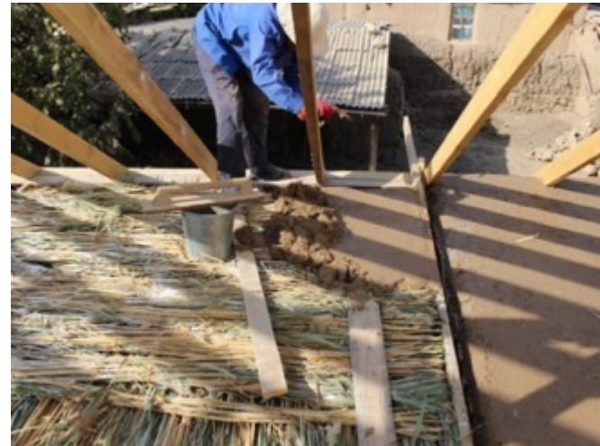
Insulation of ceiling
