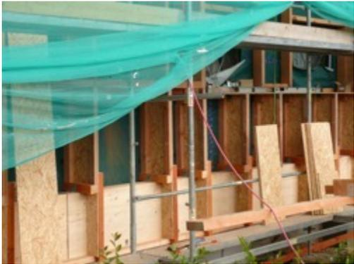
*Solution with timber frame structure, covered with wind mineral wool boards*
