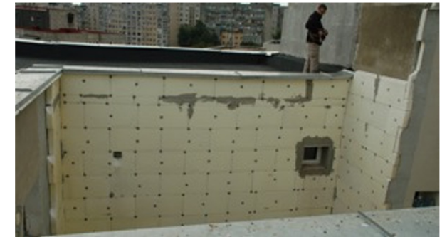
Examples with fire braking mineral wool layers
