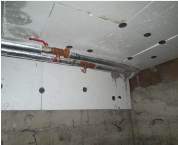
Use of EPS for cellar slab insulation Embedded wires and lighting fixtures
