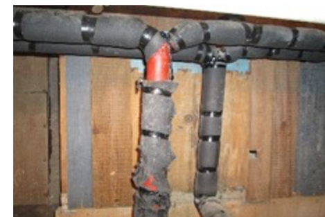
Poor quality of technical insulation
