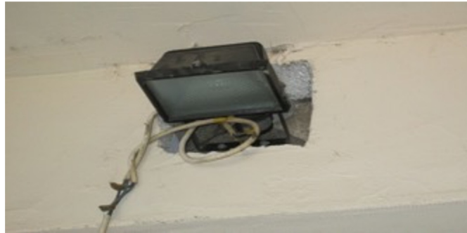
Use of EPS for cellar slab insulation Embedded wires and lighting fixtures
