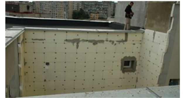
Examples with fire braking mineral wool layers
