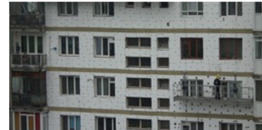
Examples with fire braking mineral wool layers
