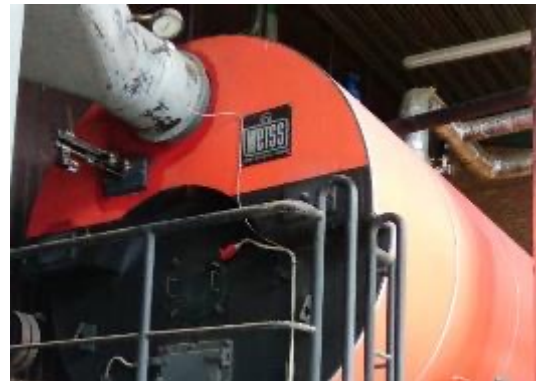
Adjustment of boilers
