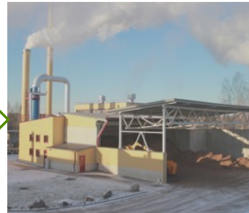
2015 flue gas condenser
