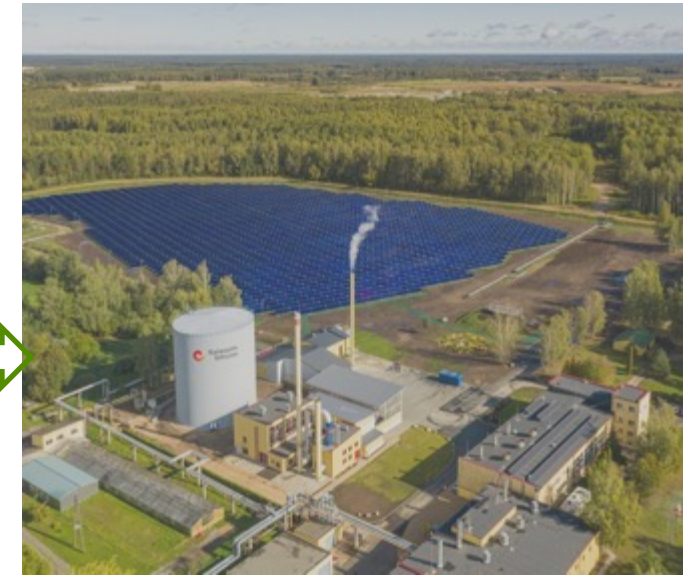
2019 1,720 solar collector field and storage tank and 3 MW wood chips boiler
